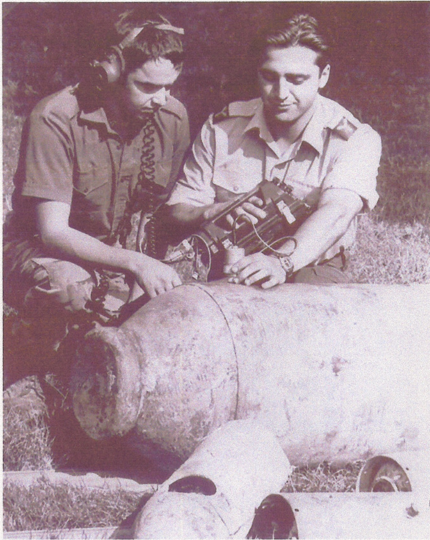
Bomb load recovered from crash site included 1 x 500 Kg and 3 x 50 Kg as seen here being worked on by the R.A.F.'s Bomb Disposal Team from Wittering. The team was led by the late W/C Keith Hopkins.
